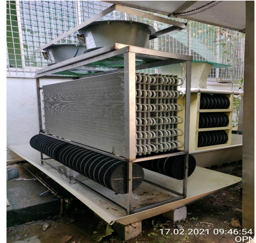
30 kW panel water heat exchanger
